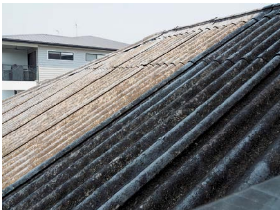
Photo 33: Close up view of single-storey east wing roof, showing typical corrugated asbestos cement sheeting used throughout all buildings.
