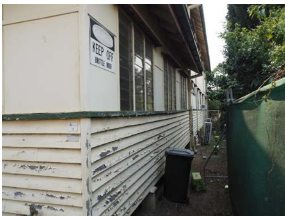
Photo 29: Northern façade (from the rear) with weatherboard linings to low level and asbestos cement linings above.
