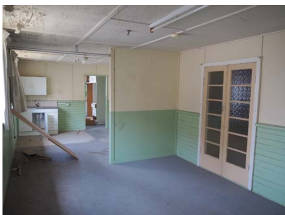
Photo 17: Typical north wing space, off the recreation hall main room. Later addition of kitchen facilities and bathroom behind (expanded hostel accommodation use). All wall and ceiling linings are asbestos cement.
