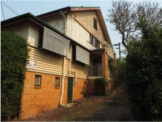
Photo 07: Main western façade facing Newdegate Street with non-original sun louvres added over glass louvre window banks.
