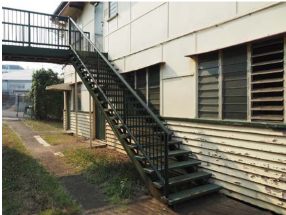
Photo 27: Southern façade access stair to upper level and bridge linking to Recreation Hall. Stair handrails non-original. Timber treads.
