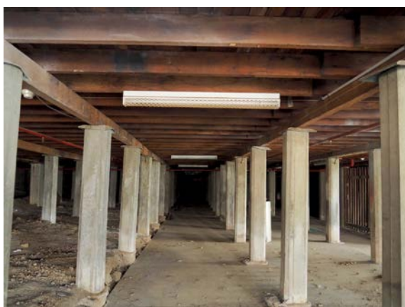
Photo 23: View of the building's underfloor concrete support columns (under recreation hall main room).
