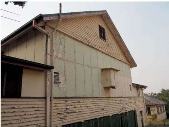
Photo 11: Rear (Eastern) façade with weatherboard linings to low level and asbestos cement linings above.
