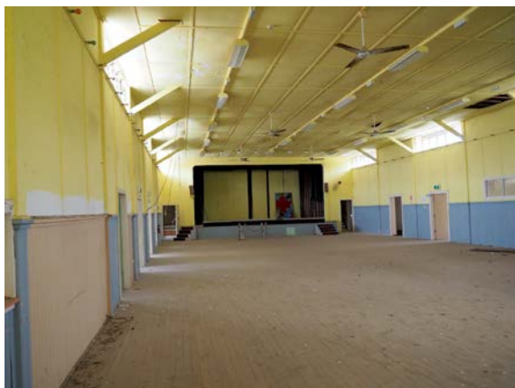
Photo 13: Recreation hall main room, looking east towards the stage with proscenium. All wall and ceiling linings are asbestos cement sheet.
