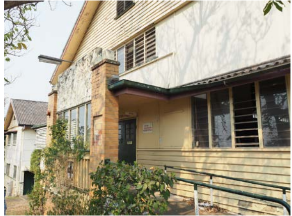
Photo 08: Main western façade facing Newdegate Street with brick entry porch in centre and non-original access ramp to right.
