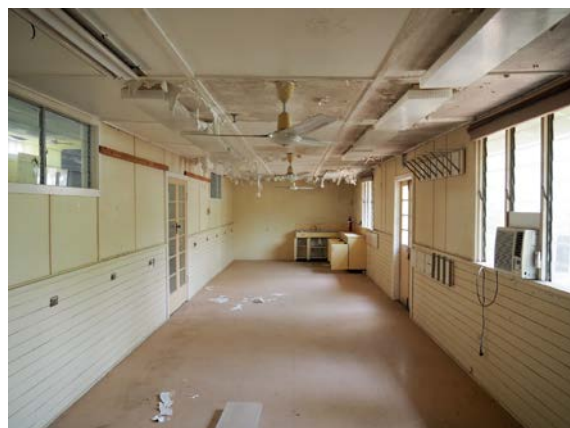
Photo 20: South wing typical room, off the recreation hall main room. Lead-based paints peeling typical. Window A/C units non-original.
