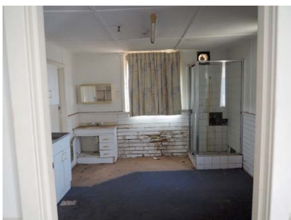
Photo 21: A more recently converted caretaker's flat in south-east corner of south wing. Issues of severe moisture, mould and rot from this incompatible use.
