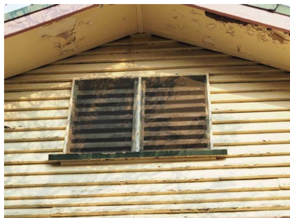
Photo 32: Timber roof vent in gable roof end to Newdegate Street western façade.
