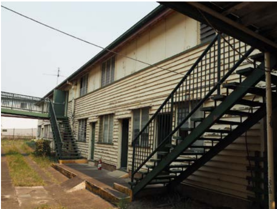
Photo 09: North wing façade with stairs leading to main hall and bridges. Stair handrails non-original.
