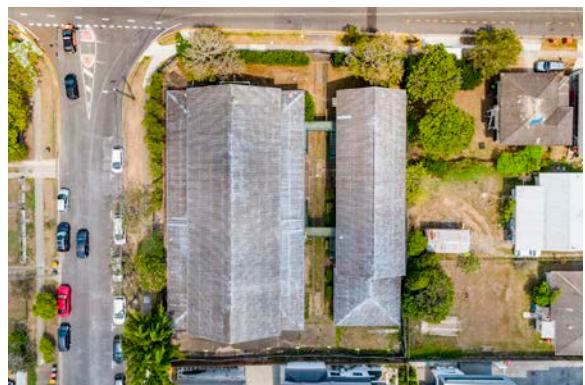
Photo 06: Drone view showing asbestos cement sheet roof profiles and link bridges. Larger Recreation Hall to the left and smaller Accommodation Hostel to the right.
